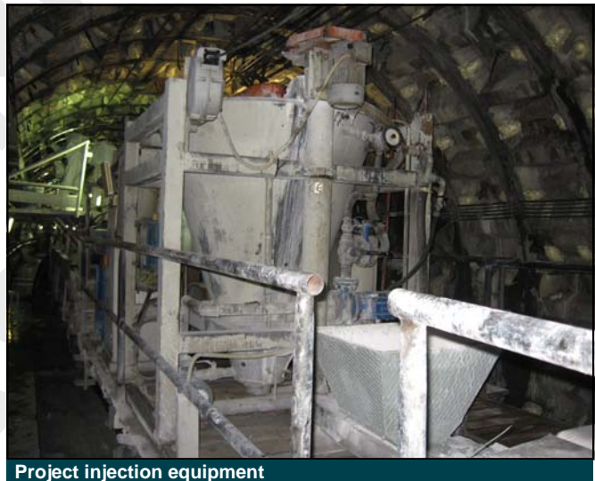
Project injection equipment
