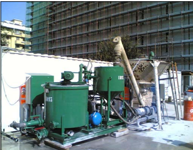
Figs. 8 and 9 - Mixing and injection system
