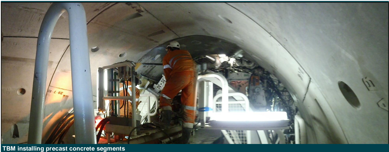
TBM installing precast concrete segments
