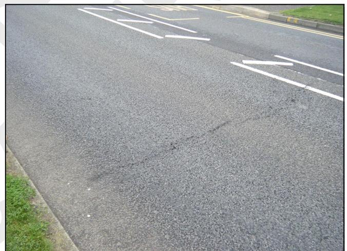
Transverse cracking apparent on unreinforced section
