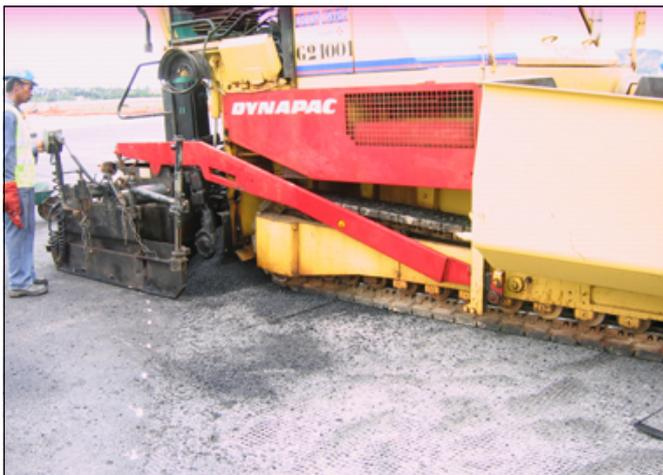
Placing of the asphalt onto the MacGrid® AR 10.7
