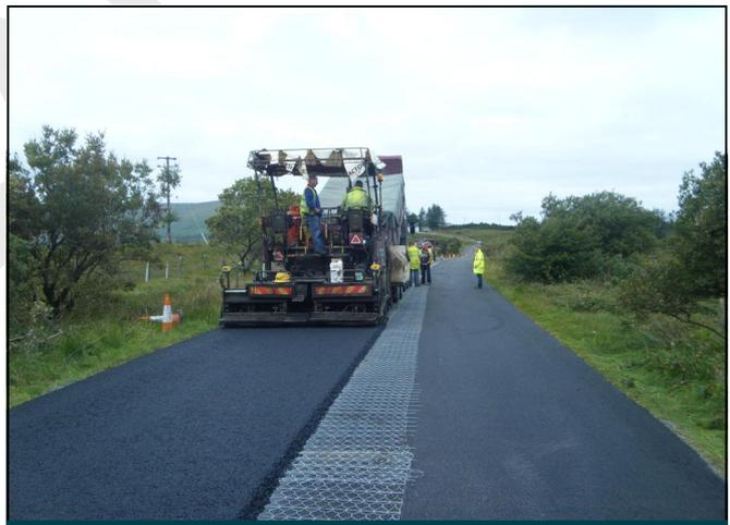
Paver running at normal speed using the 'blinding technique'
