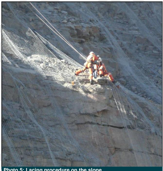
Photo 5: Lacing procedure on the slope
