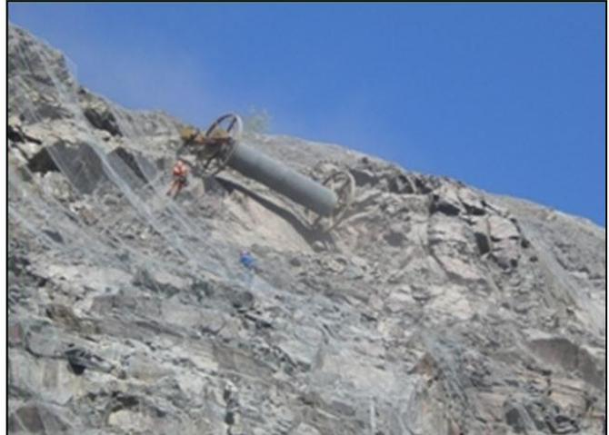
Photo 4: Installation Procedure-Decoil Machine on the slope
