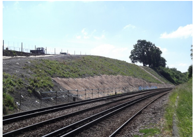
Steelgrid HR30 mesh following installation
