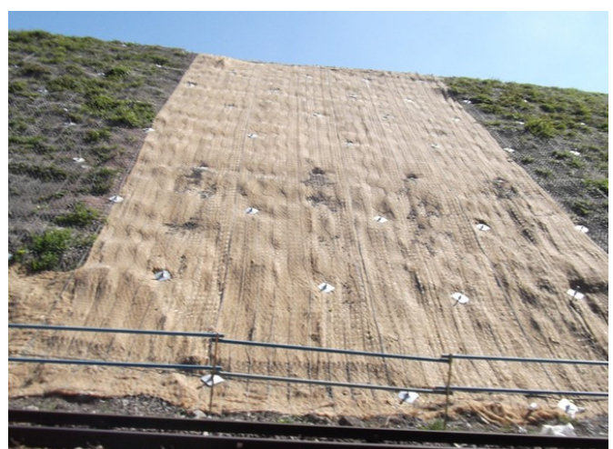
Steelgrid HR30 mesh underlain by Coir blanket
