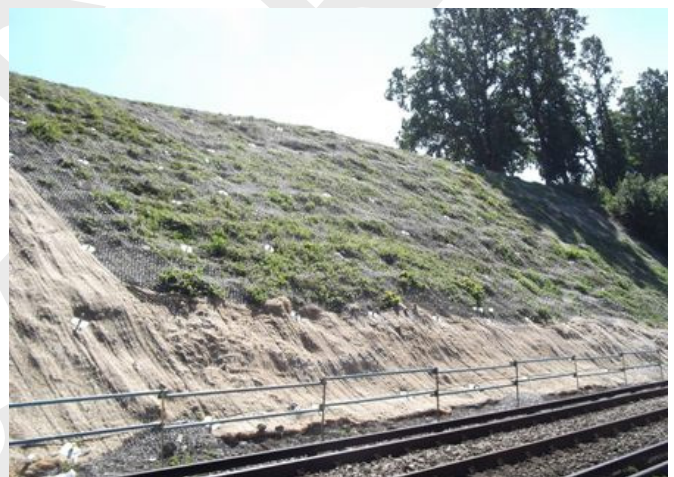
Steelgrid HR30 mesh following installation
