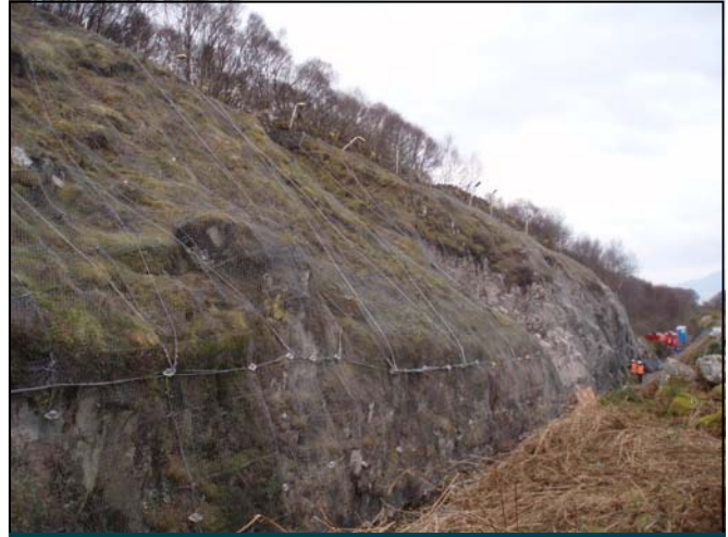
Project nearing completion
