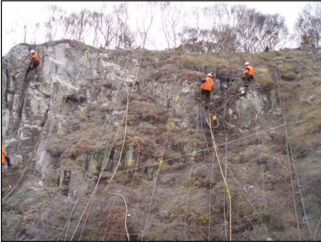
During construction using roped access specialists
