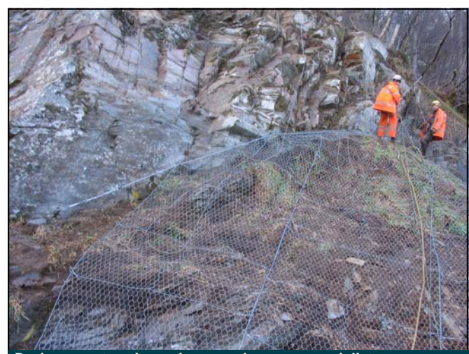
During construction using roped access specialists
