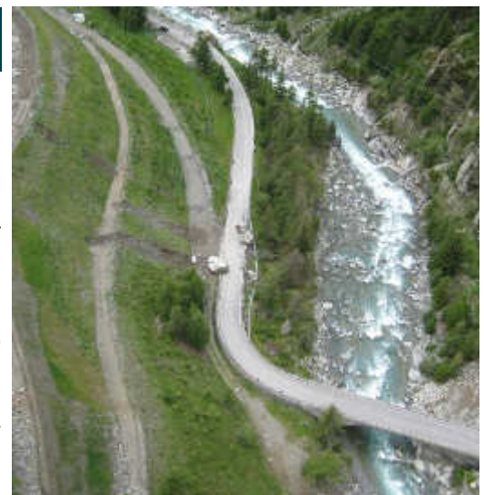
Fig 2. The post-situation, viewed from above
