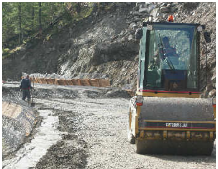
Fig 8. Compaction of lifts of fill material
