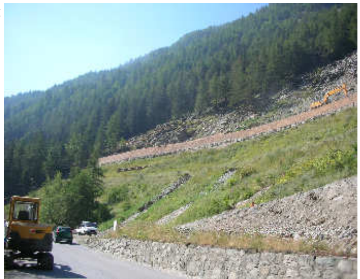
Fig 9. Embankment construction, view from downstream (SR47)
