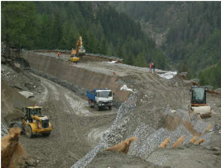
Fig 7. The embankment under construction
