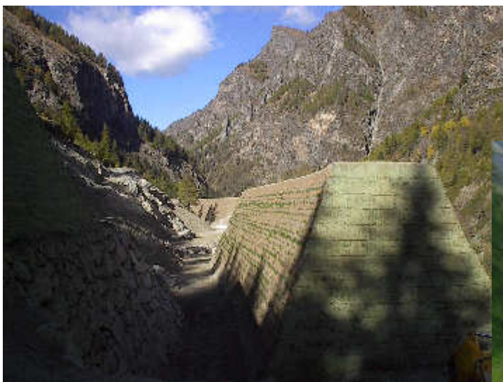
Fig 11. Lateral view of upstream embankment after completion of construction phase works.
