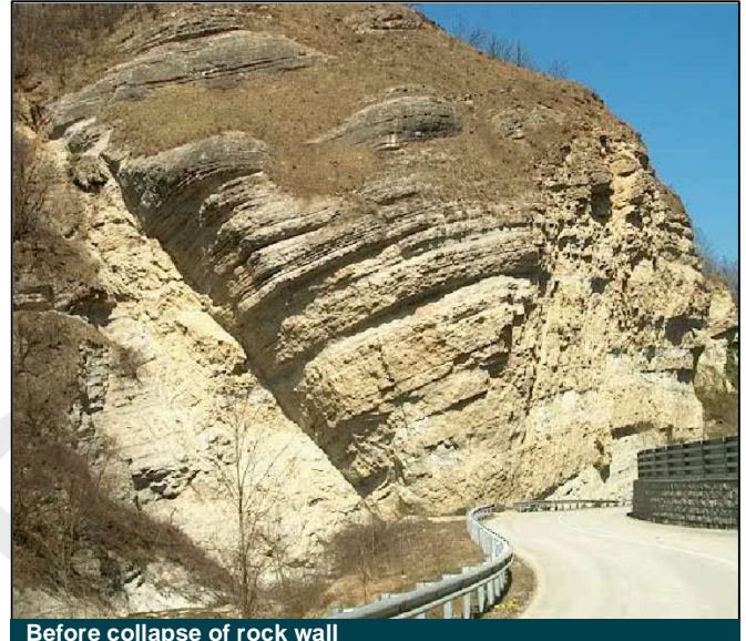
Before collapse of rock wall
