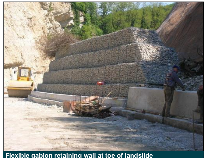
Flexible gabion retaining wall at toe of landslide
