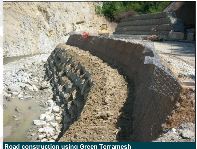
Road construction using Green Terramesh
