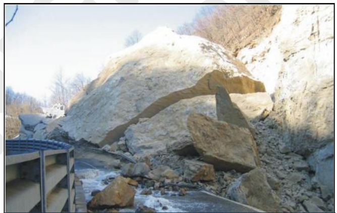
Close-up of road after collapse of rock wall
