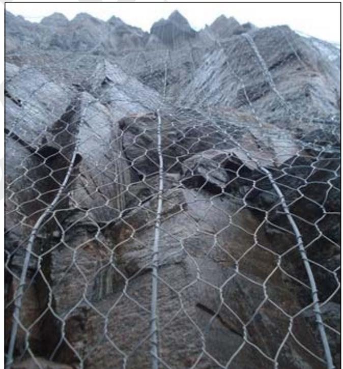
Detail of the 8 mm longitudinal cable of Steelgrid HR
