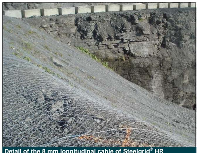
Detail of the 8 mm longitudinal cable of Steelgrid® HR
