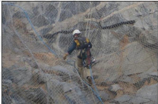
Steelgrid MO draped over face and adjacent panels connected
