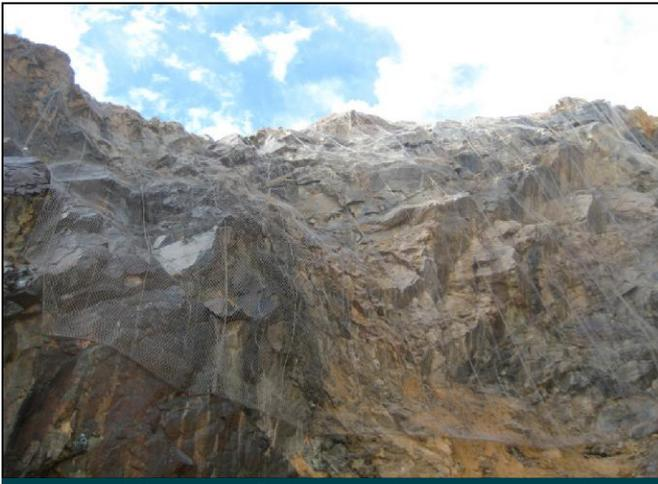
Flexibility of Steelgrid MO allows good adherence to cut face
