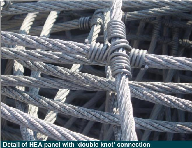
Detail of HEA panel with 'double knot' connection
