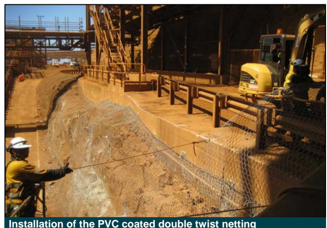
Installation of the PVC coated double twist netting
