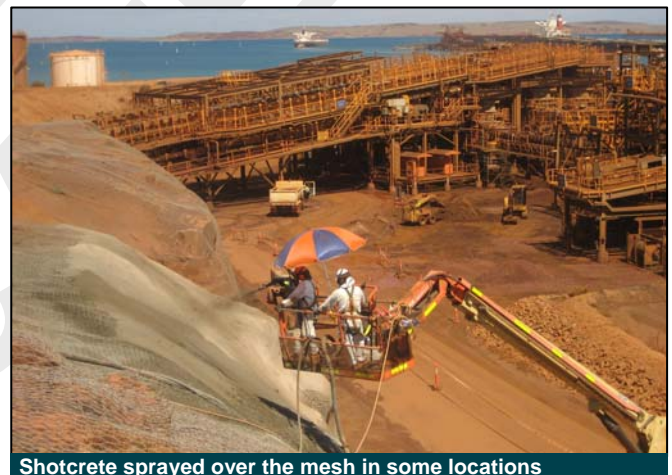
Shotcrete sprayed over the mesh in some locations
