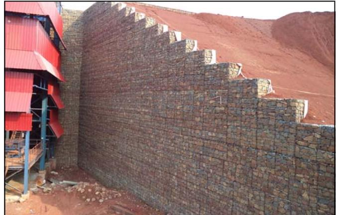
Crusher walls and wing walls that support on-site ore processing
