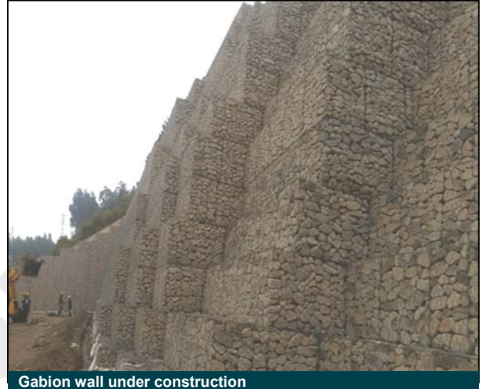
Gabion wall under construction
