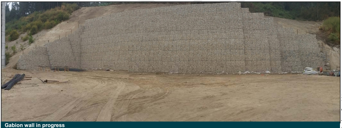
Gabion wall in progress
