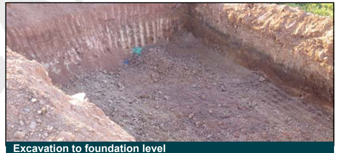
Excavation to foundation level
