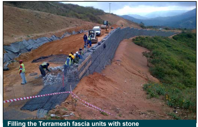
Filling the Terramesh fascia units with stone
