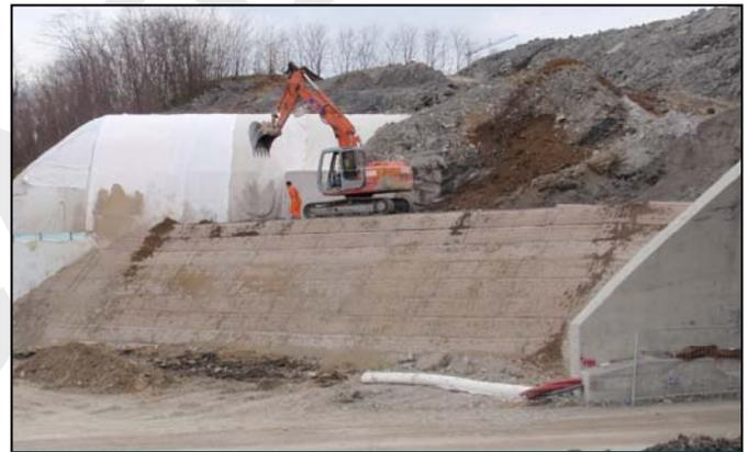
Placing backfill in zone between two tunnel portals
