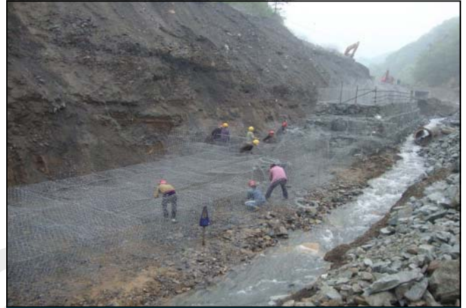
During construction of gabion walls, March 2012
