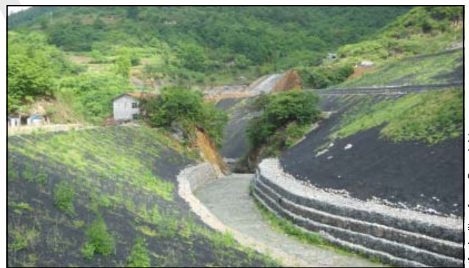
After construction, showing early plant growth, May 2013
