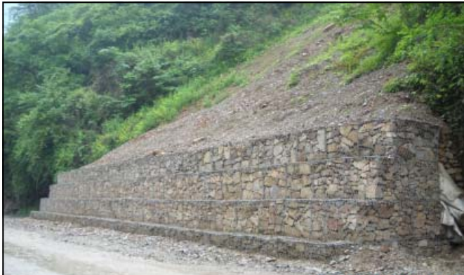
After construction, May 2013
