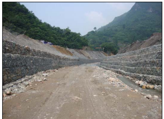
During construction, May 2012
