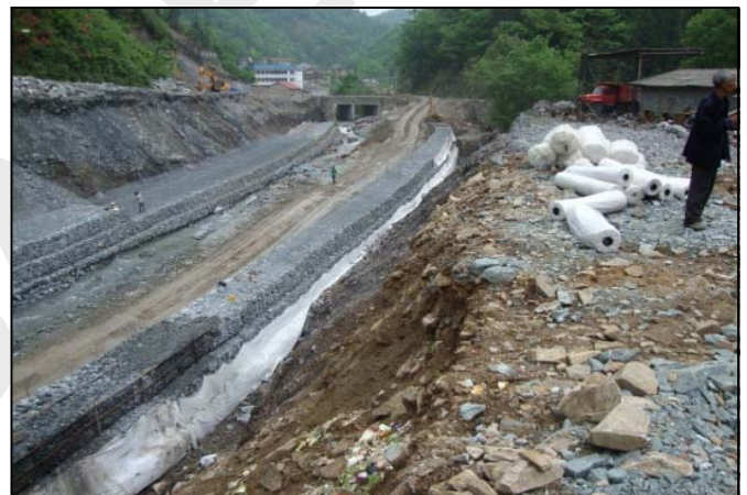
During construction, March 2012
