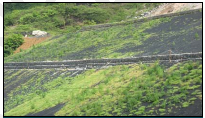
After construction, May 2013
