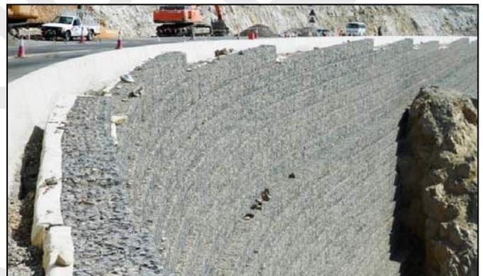
**Compaction of backfill onto Paralink geogrid reinforcement**
