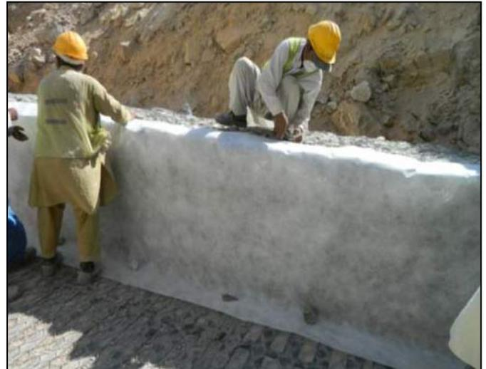
**Installation of geotextile at back of Terramesh unit**
