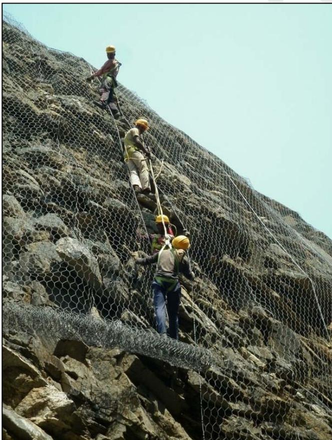
Installing the Steelgrid MO mesh onto the rock slope
