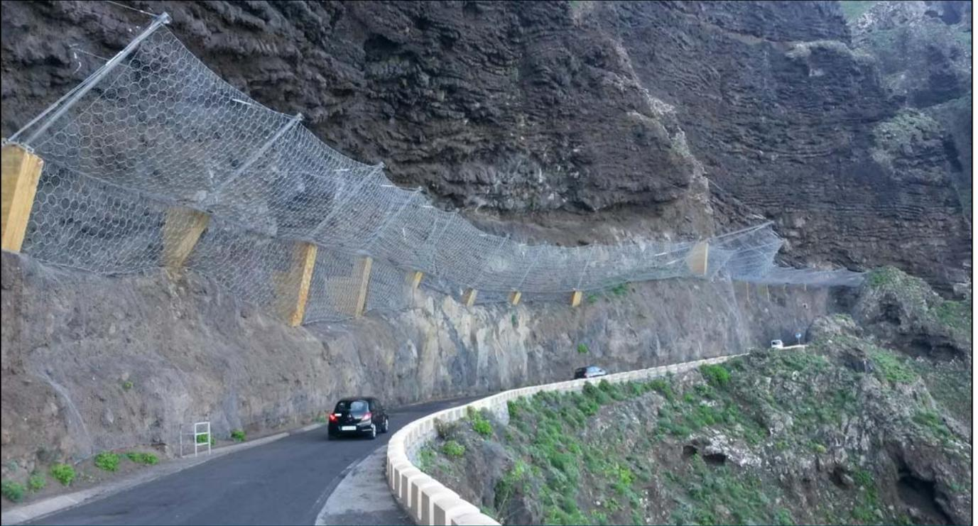
Rockfall Barrier Installed directly above the highway due to space constraints and topography of the rock face above
