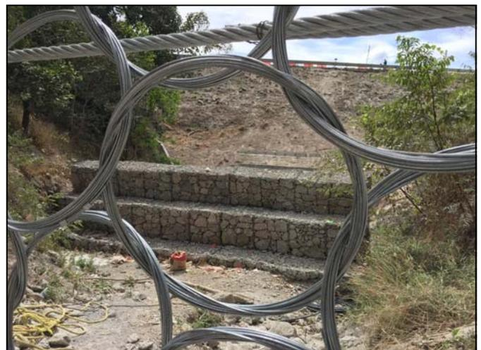
Detail of the ringnet panel of the DF Series barrier
