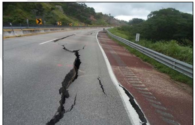
Secondary effects caused by clogged highway drainage
