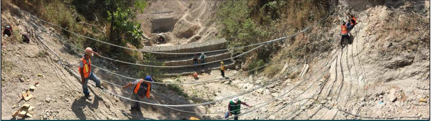
Installation of the support cables on either side of the chute
