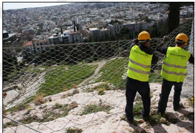
During 250kJ Barrier Installation
