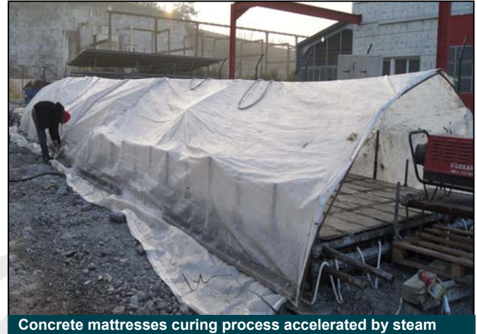
Concrete mattresses curing process accelerated by steam
