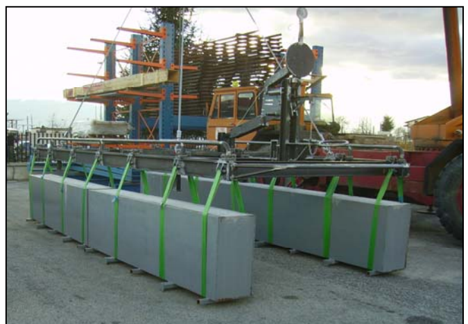
Loading test on an ROV automatic frame suitable for deep water ACBM launching operations
