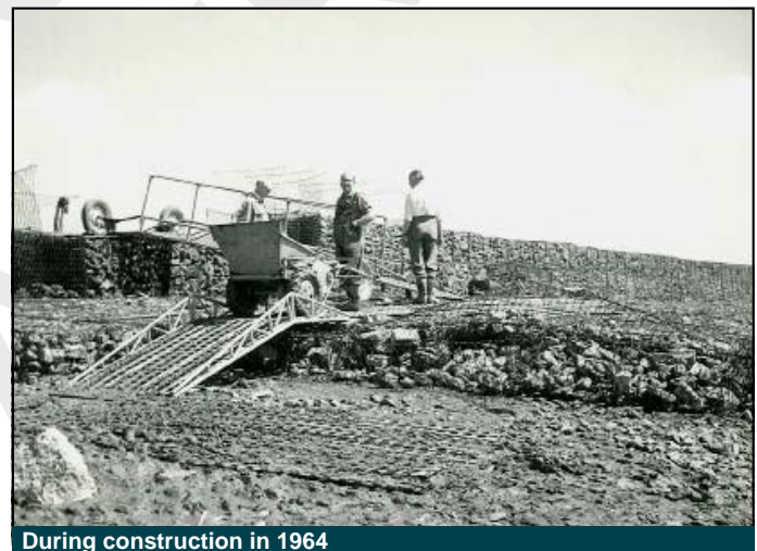
During construction in 1964
