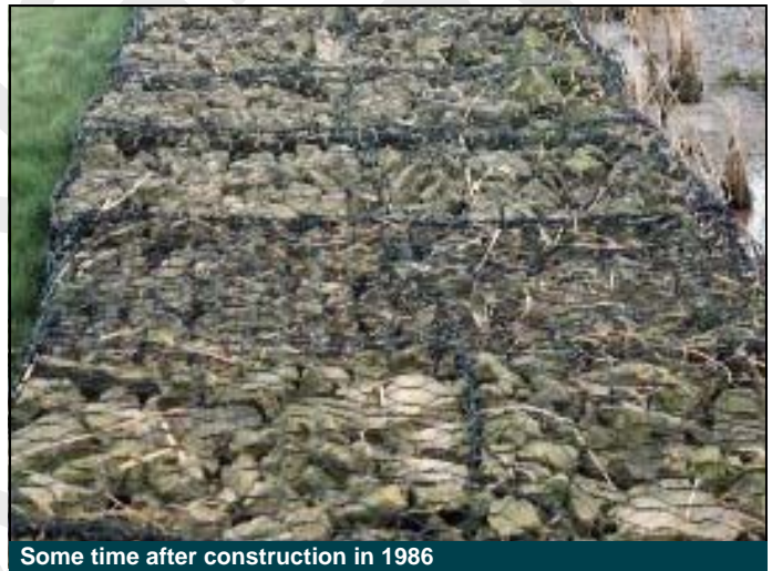
During construction—showing nature of erosion
