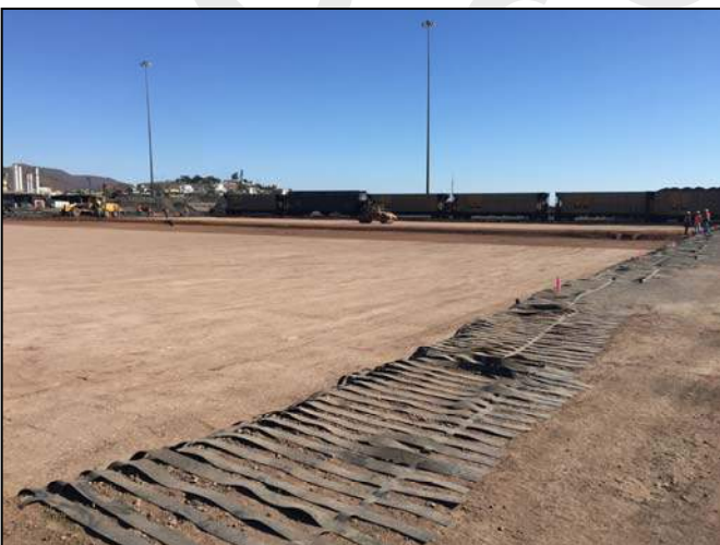
Final stage of ParaLink installation
