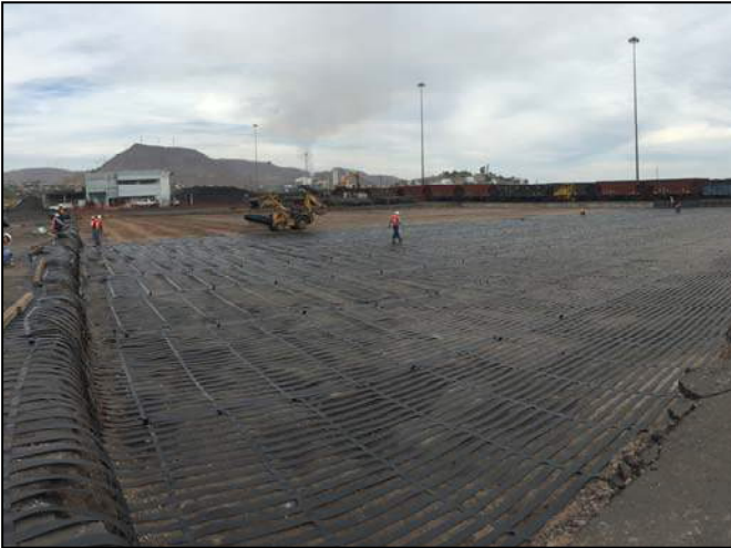
ParaLink® 600 first layer installation
