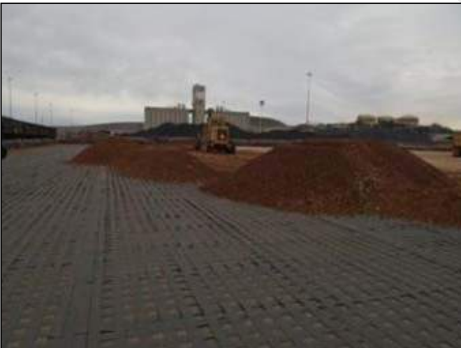
Placing filling material
