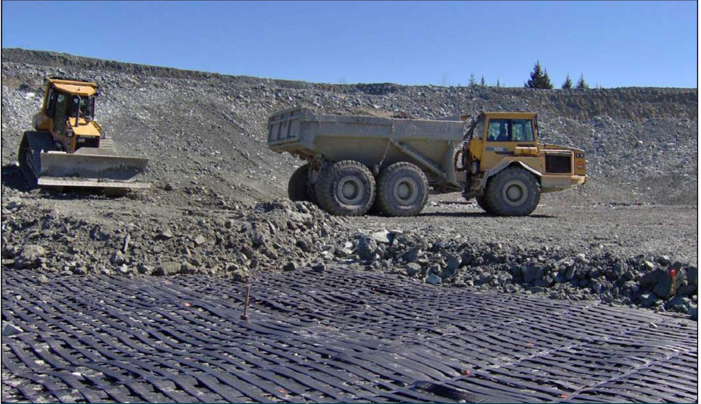
Placement of structural backfill directly on top of Paralink®
