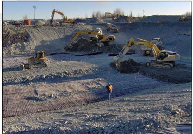
Structural backfill nearing completion
