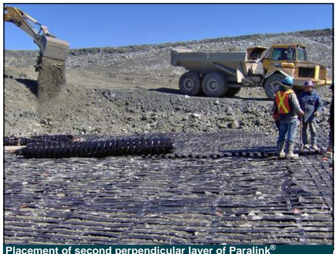
Placement of second perpendicular layer of Paralink®
