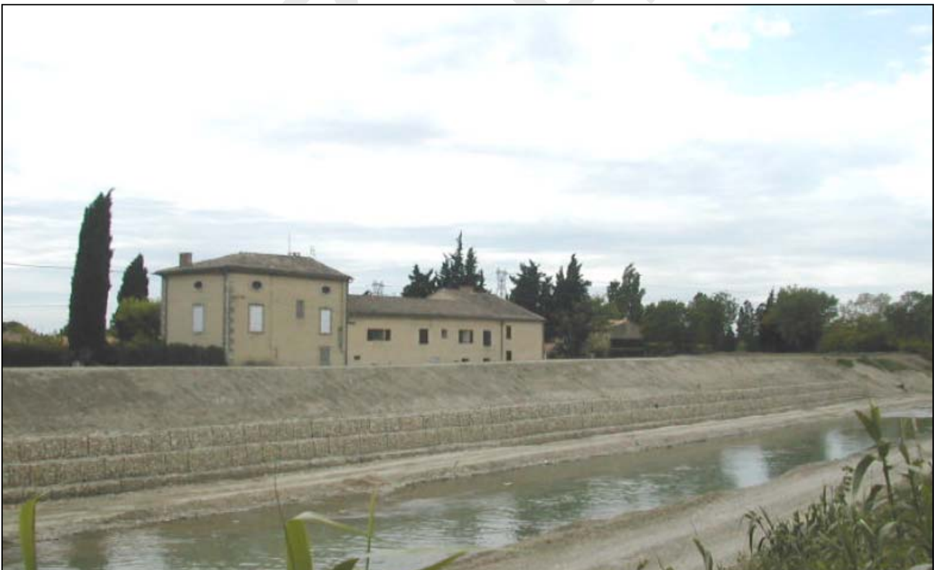
Completed installation, immediately after completion of works
