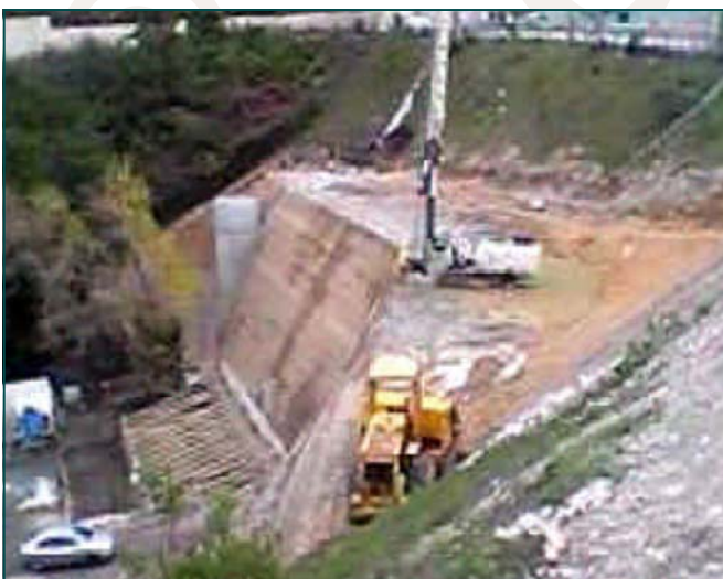
During construction (future cell containment wall)
