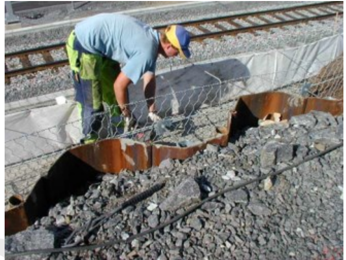
During the construction
