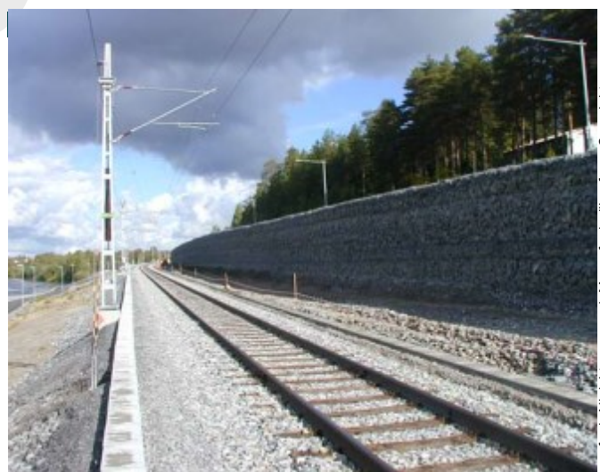
After the Construction
