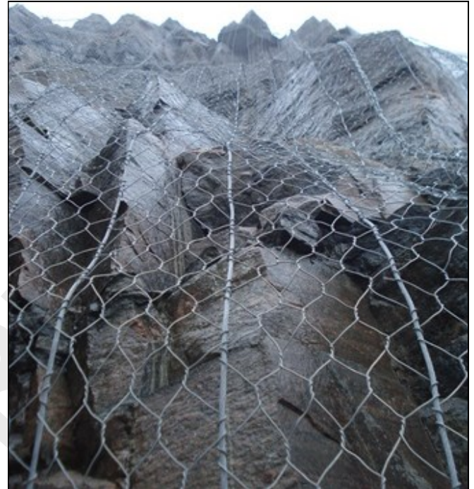
Mesh runs hanging during installation
