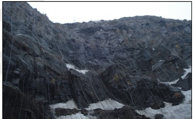
Slope topography overhung by mesh during installation
