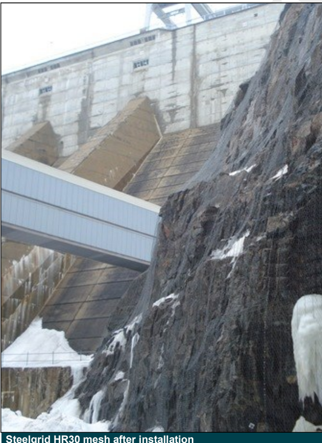
Steelgrid HR30 mesh with ice accumulation
