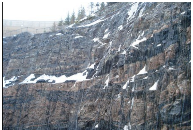
Mesh conforming to slope topography after installation
