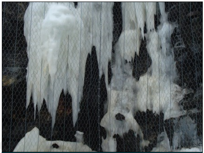
Steelgrid HR30 mesh with ice accumulation
