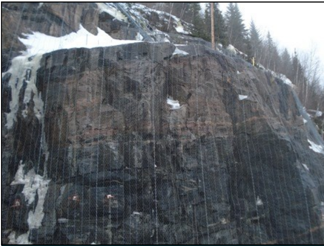
Steelgrid HR30 mesh after installation
