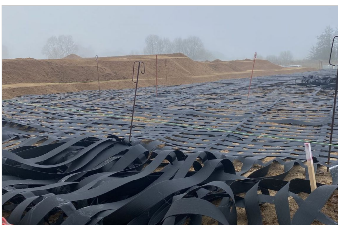
Detail of the overlapped grids in perpendicular direction
