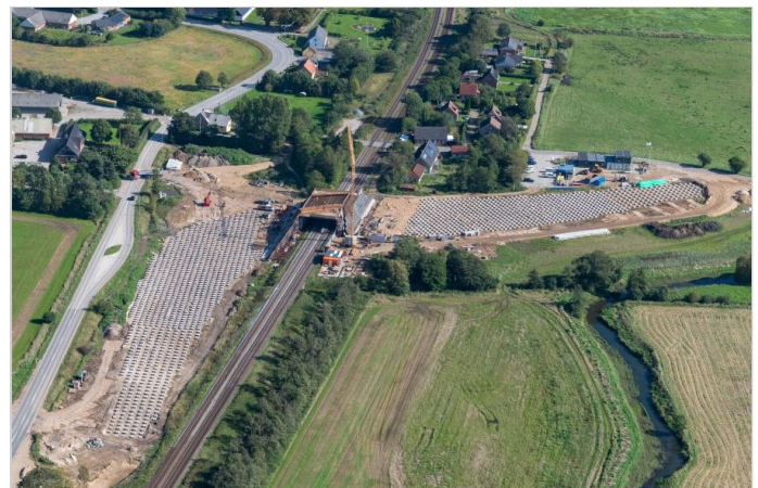
Drone aerial view of the pile caps
