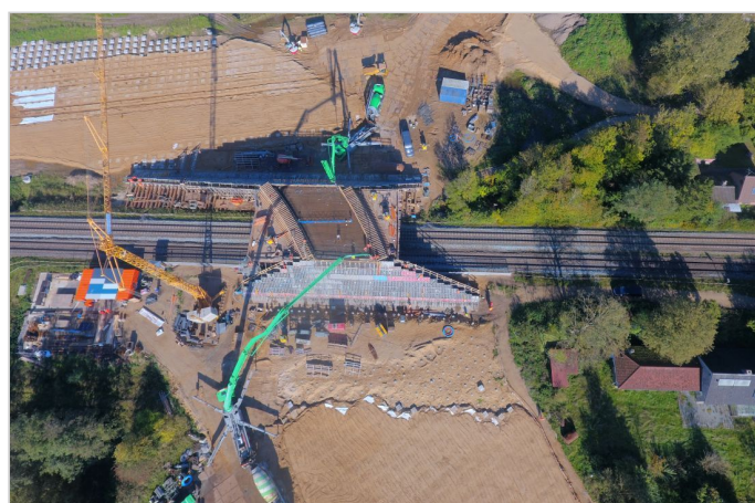
Drone aerial view after the covering of the pile caps
