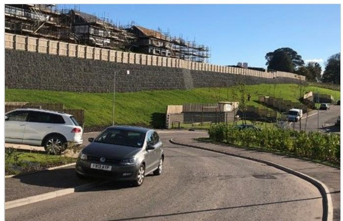
Long distance view of the Terramesh® system with fence
