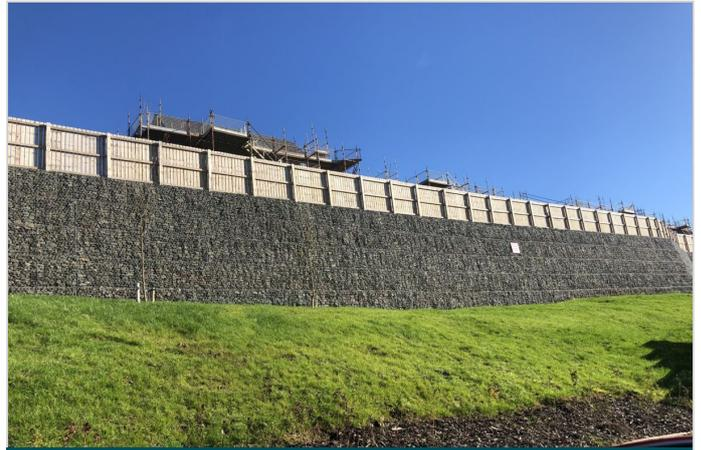
Gabion wall complete with fencing on the top—just over 5m tall retaining wall
