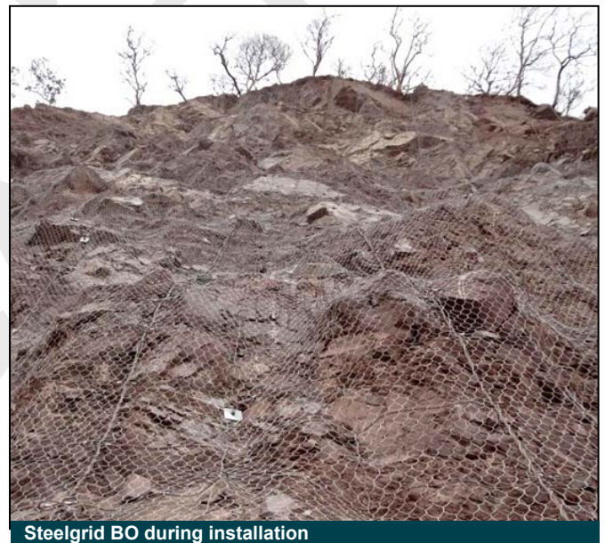
Steelgrid BO during installation
