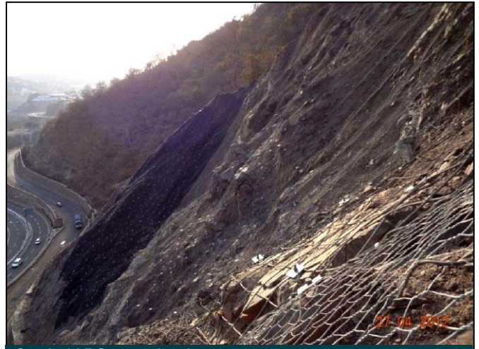
Steelgrid BO on rocky slope
