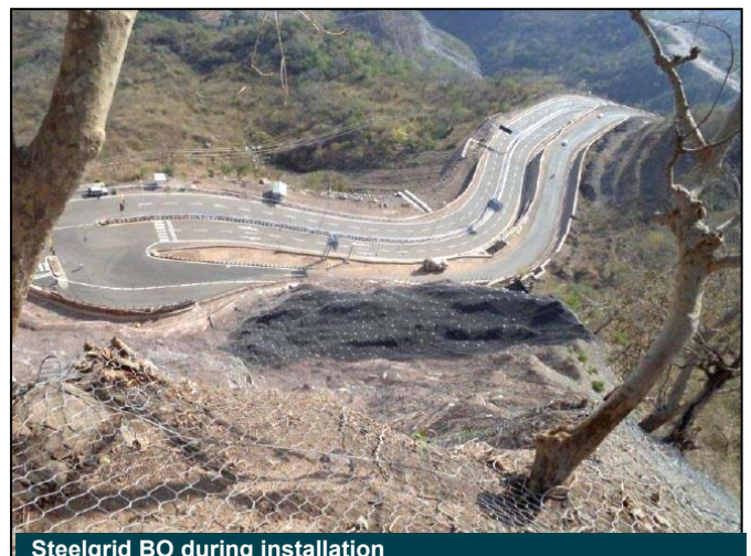
Steelgrid BO during installation
