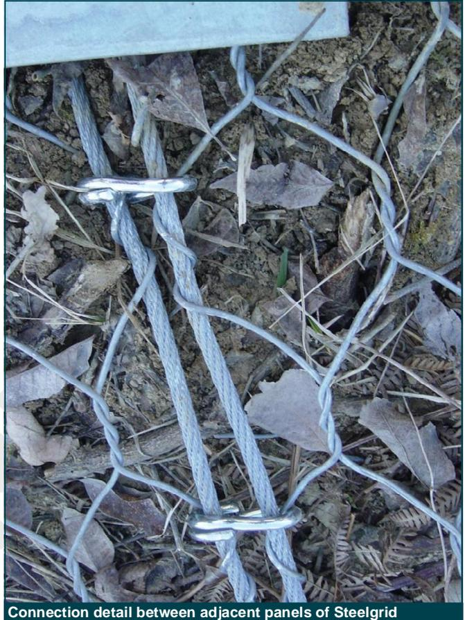
Connection detail between adjacent panels of Steelgrid
