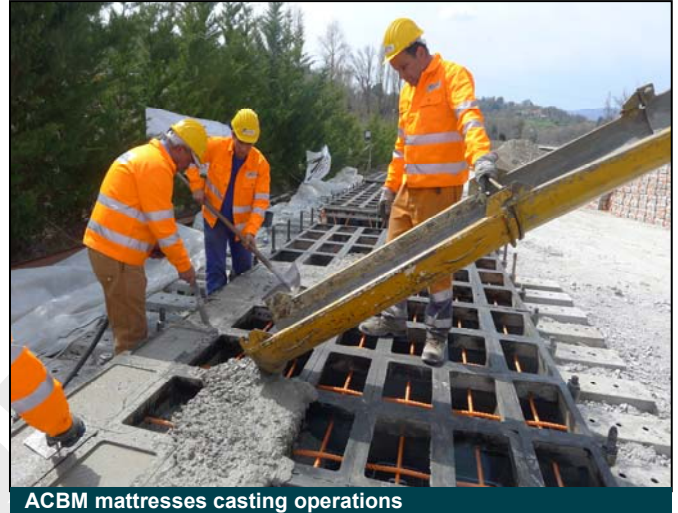
ACBM mattresses casting operations
