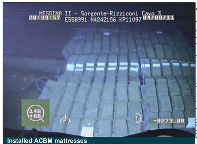
Installed ACBM mattresses
