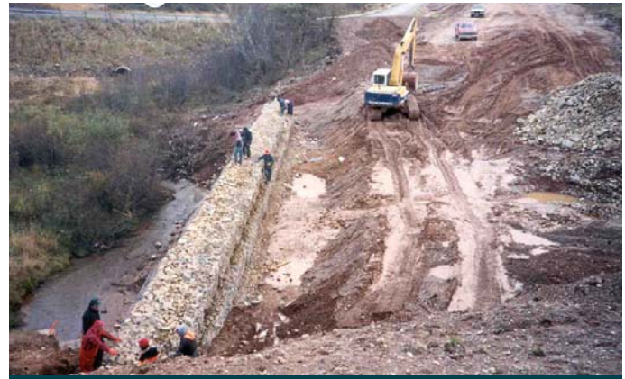
Original Gabion Retaining Wall under construction, 1990
