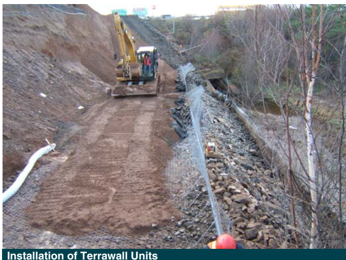
Installation of Terrawall Units
