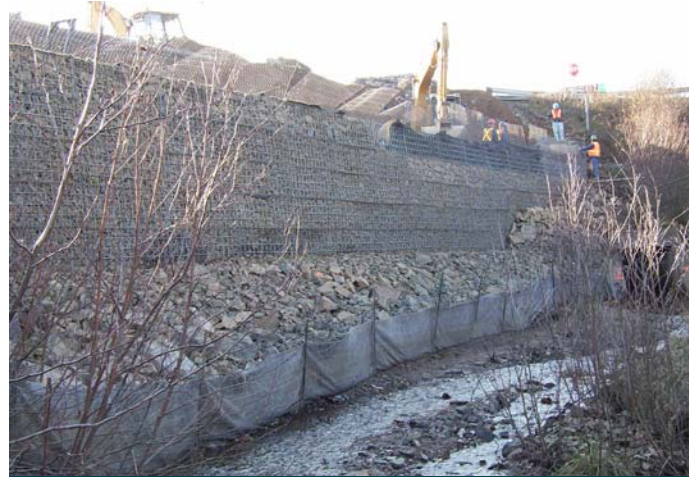
Terrawall Structure partially completed
