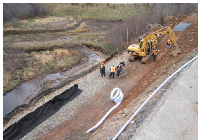
Foundation Terrawall Units being installed
