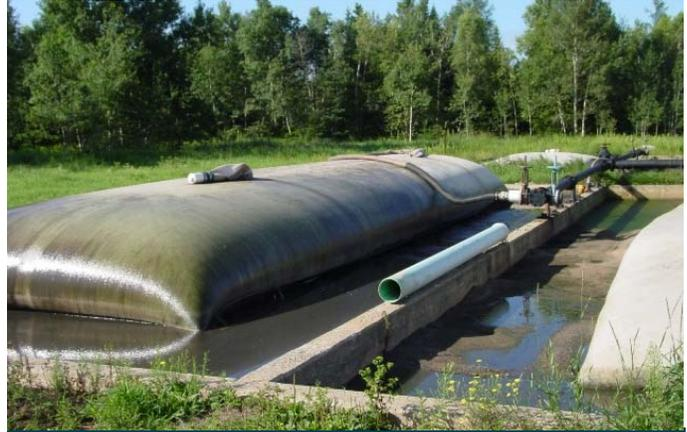
MacTubes™ connected via manifold to Treatment Plant
