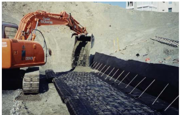
Foundation of Terrawall w/ ParaGrid 200/15
