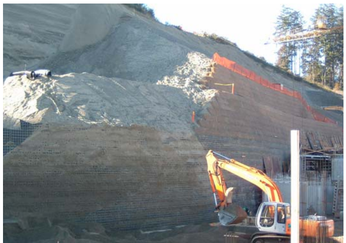
Completed Terrawall w/ Green Terramesh under construction
