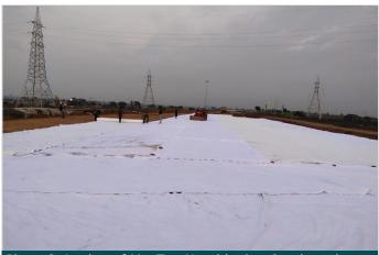
Photo 2: Laying of MacTex N at blanket & subgrade interface
