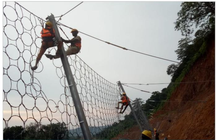
Figure-4 Installation of Primary Interception mesh (MacRing)
