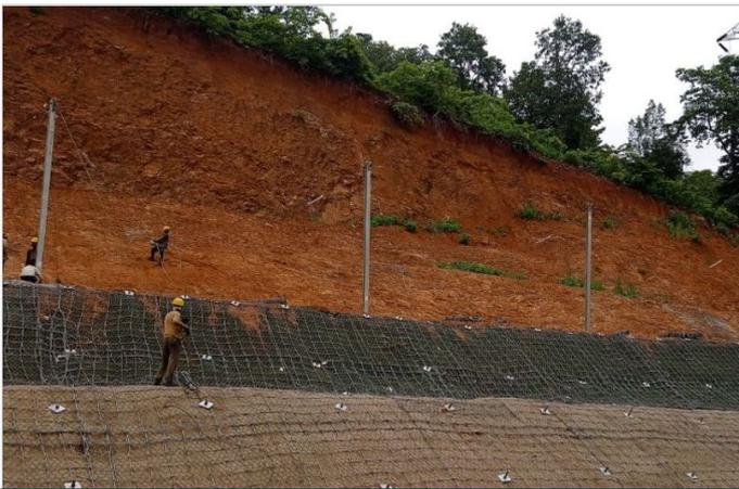
Figure-3 Connecting upslope or lateral anchors with help of bracing cables
