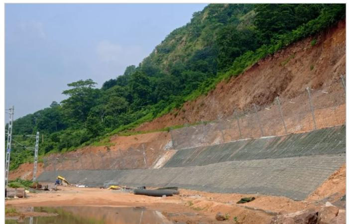
Figure-6 Overall site after the installations of Rockfall barriers
