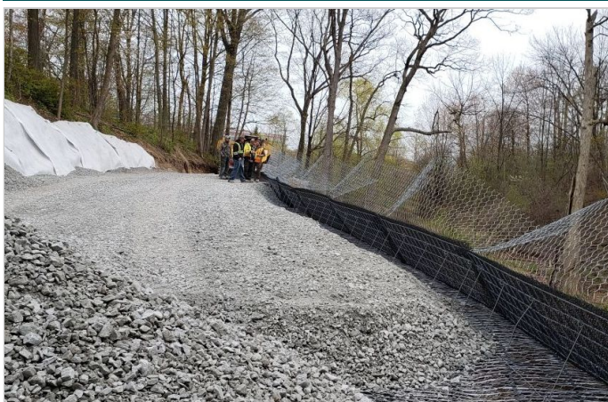
Free Draining Granular Backfill with ParaDrain
