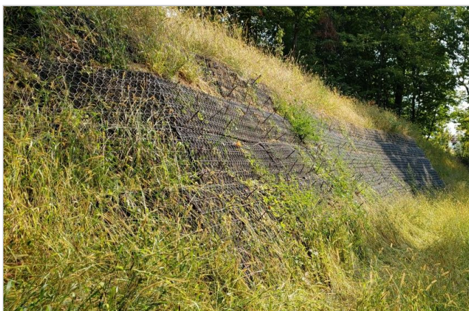
Completed Green Terramesh Slope
