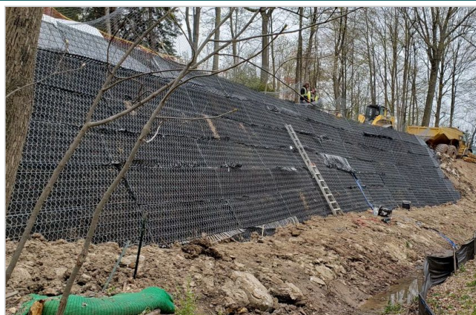
Partial Green Terramesh Installation
