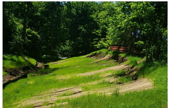
Failed Slope with Temporary Erosion Control Blanket
