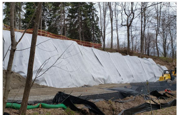
Start of Construction - Cut Slope with MacDrain Installed
