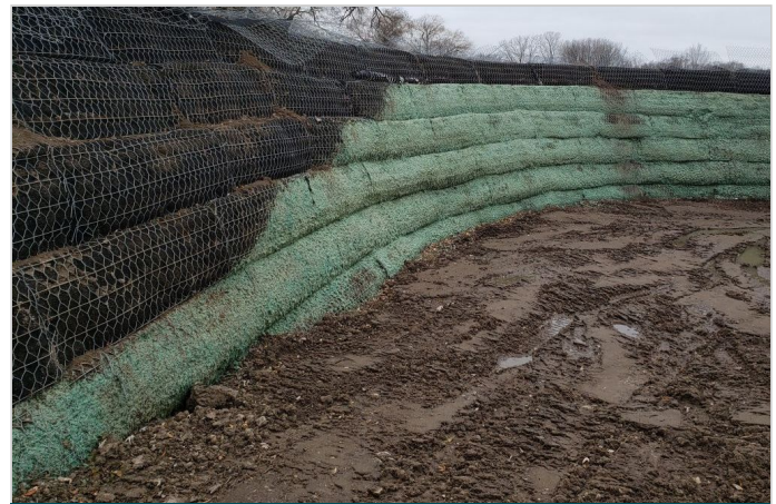
Detail of hydroseeding over Green Terramesh
