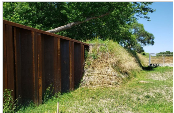
Detail of finished Green Terramesh wrapping sheet pile wall
