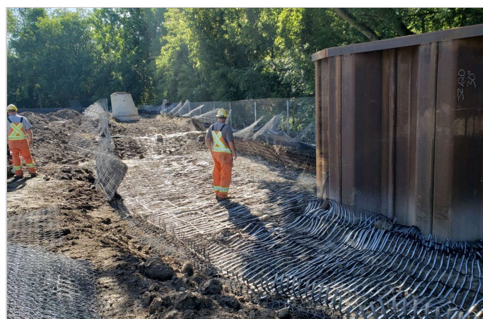
Detail of Paradrain placement during construction of Green Terramesh
