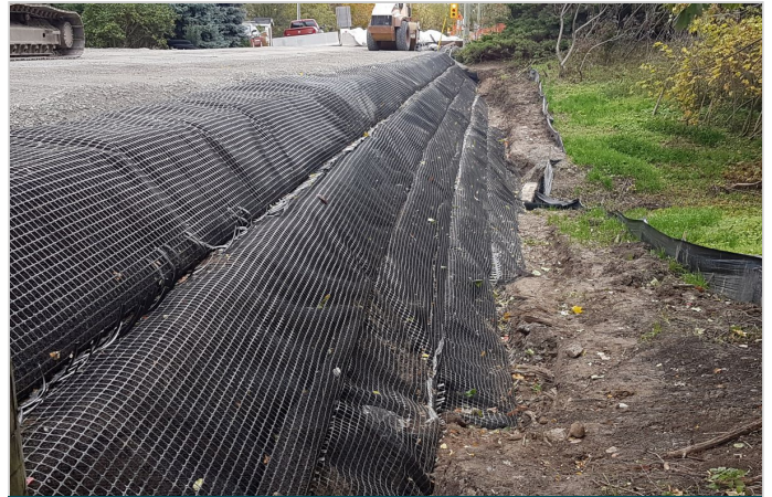
Reinforced slope during compaction
