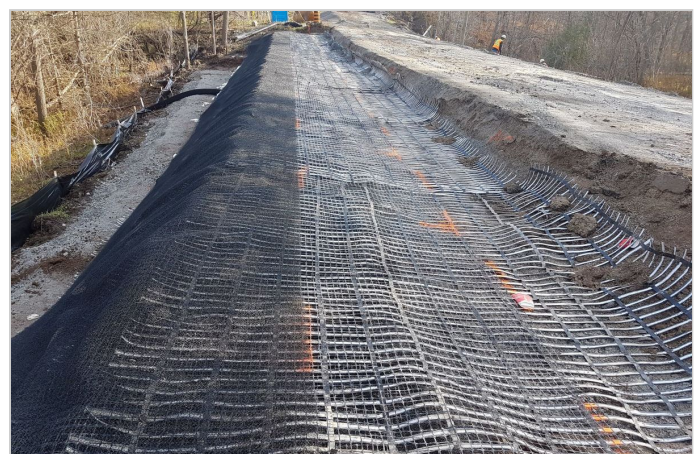
Detail of ParaDrain installation
