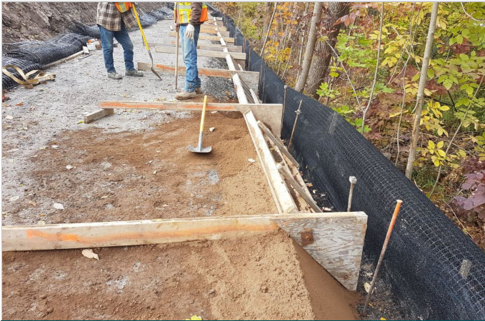
Detail of form used for wrapping
