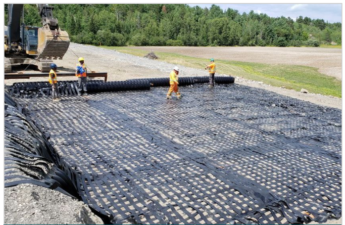
Biaxial Configuration of Geogrid Showing Overlaps
