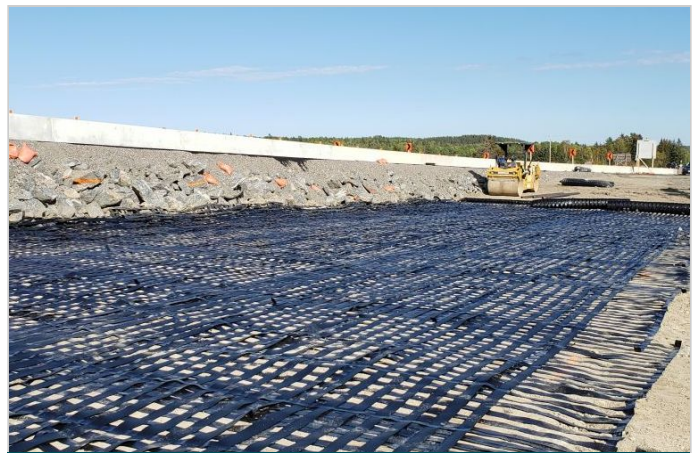
Geogrid Ready to Backfilled
