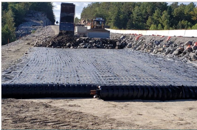
Backfill Operation using Large Angular Rocks
