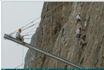
Figure 4- Installation of dynamic rockfall barrier
