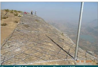
Figure 2-HEA Panels laid over Steelgrid MO on slope
