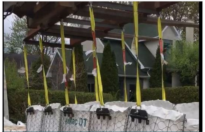
FlexMac DT unit lifting operation
